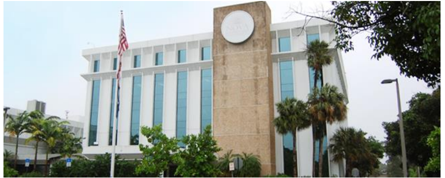
Front of East Campus Administrative building
